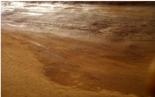
(b) A completely broken down portion of the road alignment at Isinigbo.
