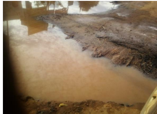
(d) An intensely eroded surface exposing the subbase and subgrade at Ikere-Ekiti.
