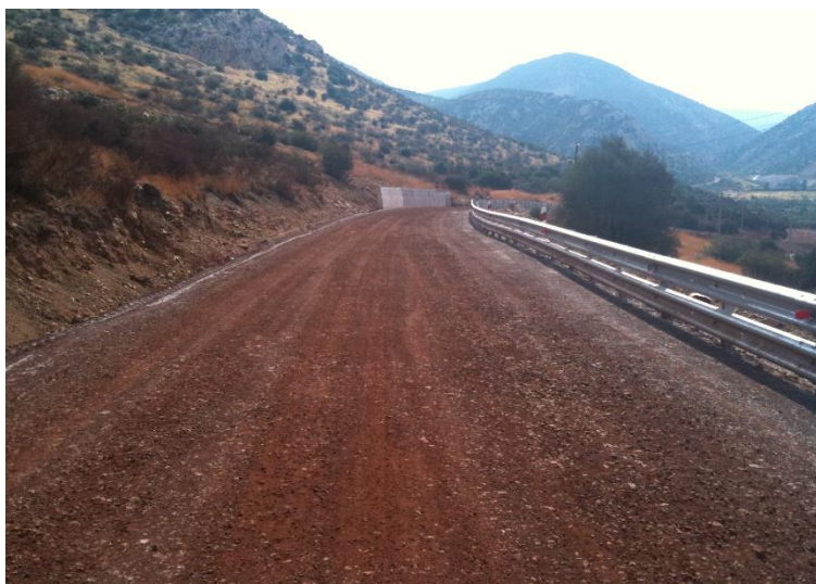
Fig. 3 The gravel road by bauxite residue.
