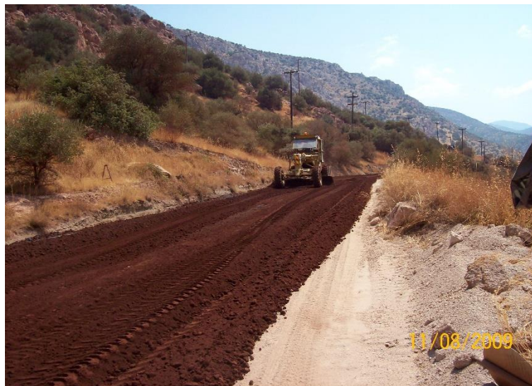
Fig. 2 The construction of the road.
