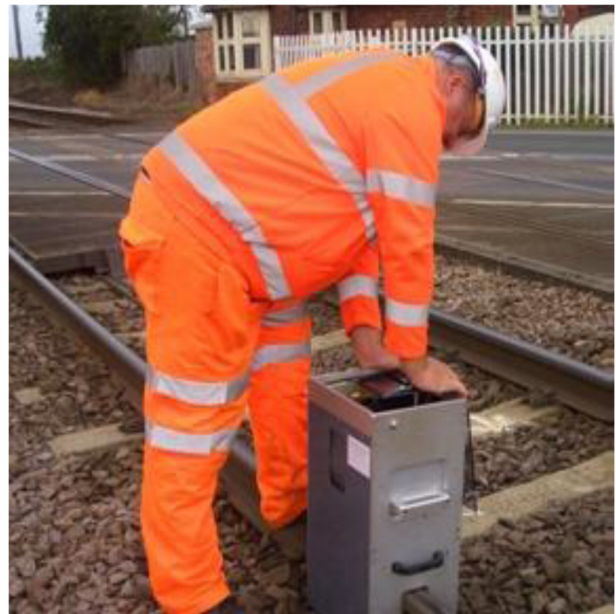
Fig. 5 G-Scan equipment being used to inspect a level crossing, the work is carried out in 'Red Zone' conditions with both road and rail open to traffic.
