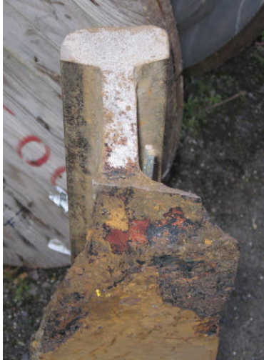
Fig. 1 Corrosion of the rail foot commonly found within level crossings with little or no loss in rail depth.
