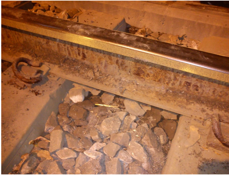
Fig. 7 No significant corrosion of the rail at Mansfield Road level crossing.
