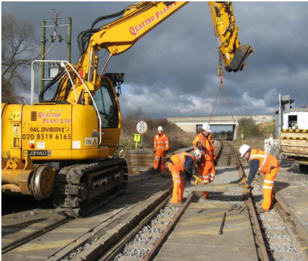
Fig. 3 Lifting the deck to allow visual inspection of the rail.
