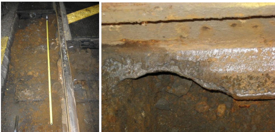
Fig. 9 The corroded section, at between 8.9m and 16.5m on the A-Scan result shown in Fig. 8, was then verified using VT showing severe corrosion of the toe section of the rail.
