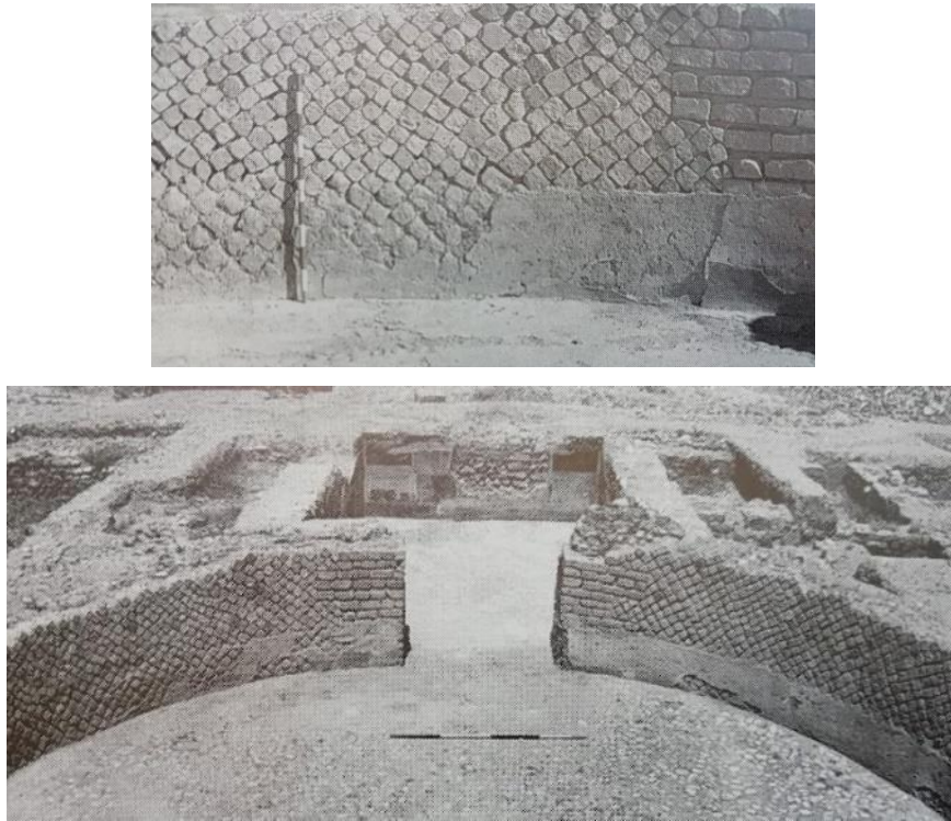
Figure 11. Examples of opus reticulatum and opus quadratum in exedra B64 (Netzer, 2001a, p. 243, Photographs 363 and 364).
