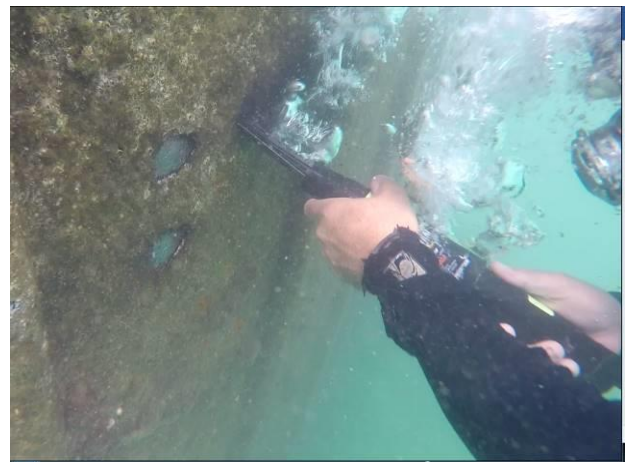
Fig. 4 Underwater cleaning of measurement points.
