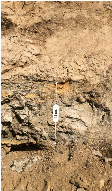
Fig. 3 The clayey filling material of the fault 26/54 F at the left side of the slope.
