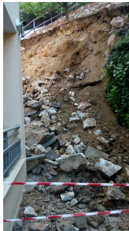
Fig. 2 A part of the landslide.
