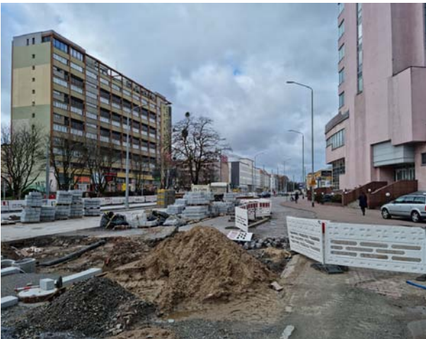
Fig. 3 Road refurbishment works at the Rodla Square in Szczecin (15.02.2022).
