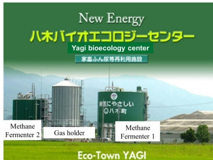
Fig. 21 Biogas production from livestock waste and food waste by methane fermentation.
