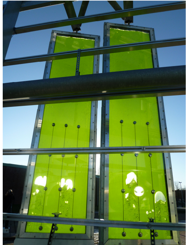
Fig. 9 Detail of Solar Leaf panels with algae [©Arup].
