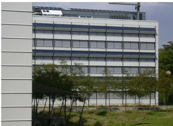
Fig. 4 View of Fraunhofer Institute building with PV components over the windows and on the roof of southern wing (Müjde Altın, August 2006).
