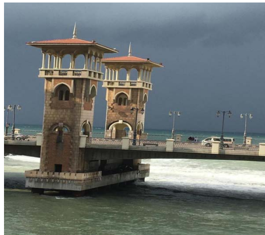
Figure 7. Towers of Stanley Bridge.
