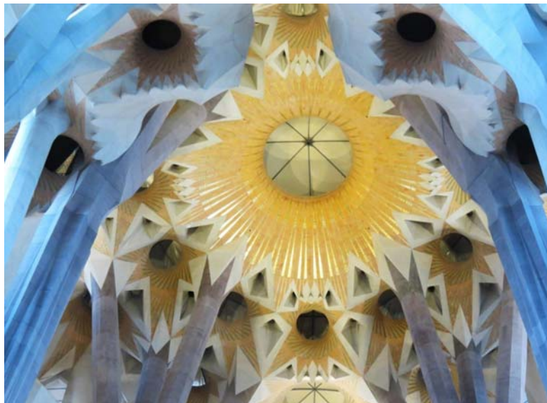
Fig. 8 Internal image signaling the rotating hyperboloids in the connecting part of the existing pillars in the Templo Expiatorio de la Sagrada Familia.
