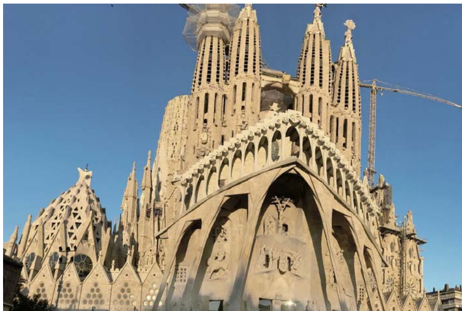
Fig. 10 External view of the church.
