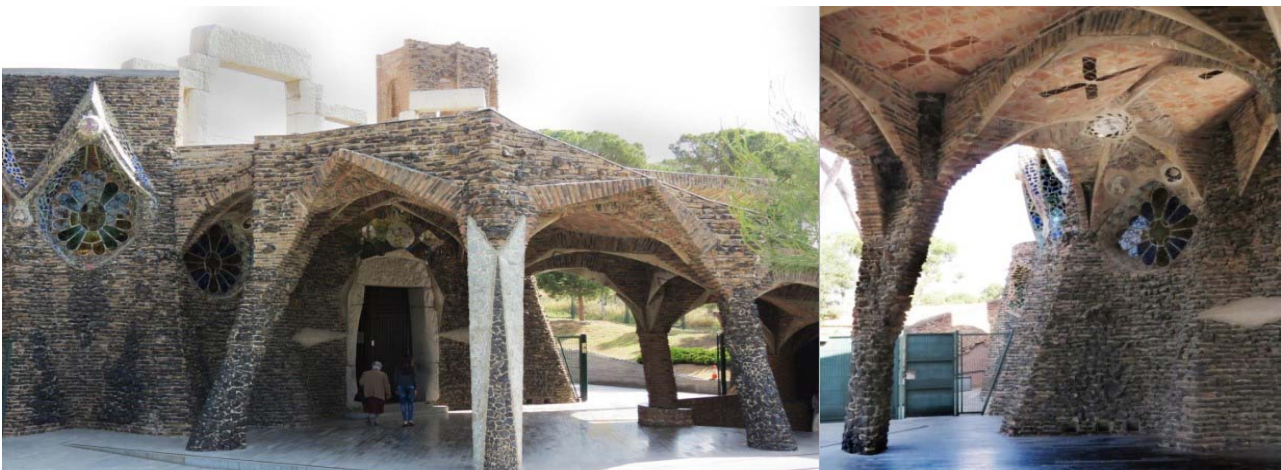
Fig. 6 (Left) external view referring to the main entrance of the crypt; (right) image showing the structural elements in catenary arches between the pillars and the main wall; and the vaults in hyperbolic paraboloids.
