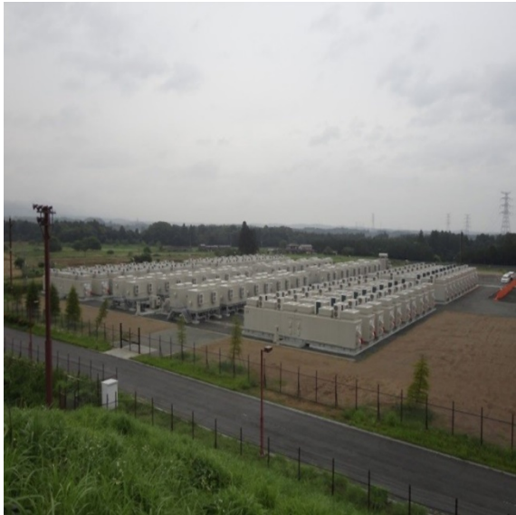
Fig. 13 Power conditioners and step-up transformers are arranged between the storage batteries lined up on both sides [31].
