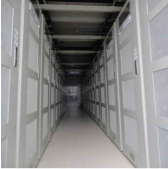
Fig. 12 Each container houses 26 storage battery panels [31].
