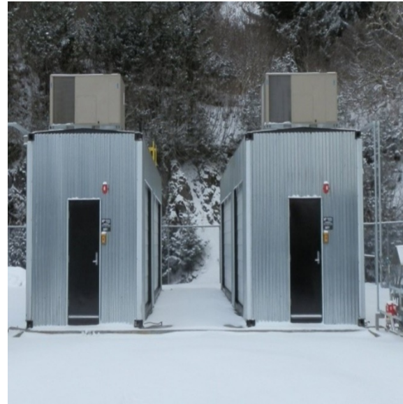
Fig. 22 Two containers housing the 3 MW / 0.75 MWh battery park on Kodiak [72].
