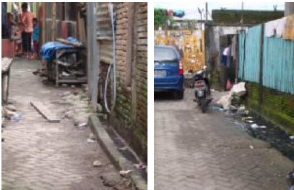
Fig. 5 Gutter and footpath: the narrowest and shallowest sewer in the settlement, this condition can not accommodate the volume of dirty water environment.
