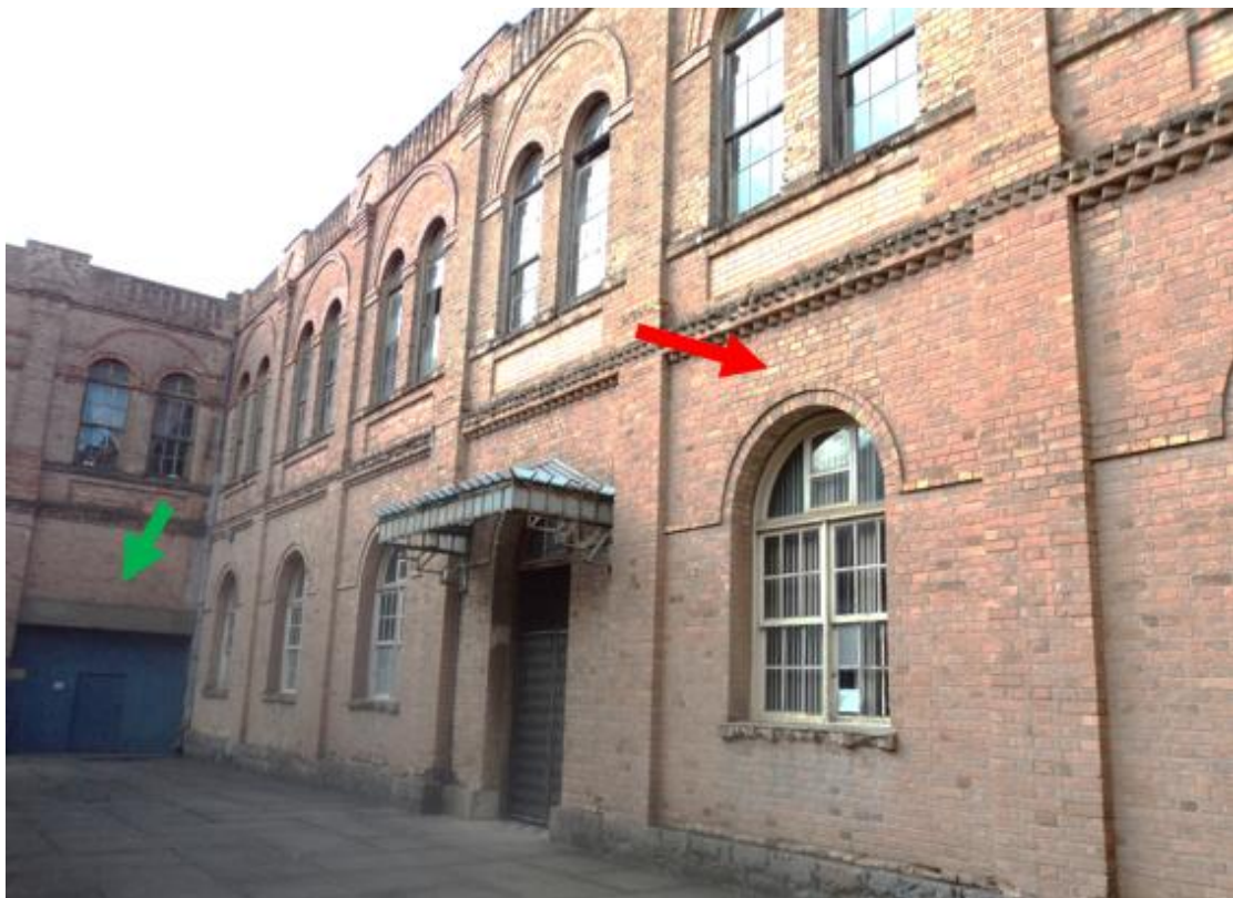
Fig. 6 Continuation of the stretch extended in the 1950s. Note the mark of the extension from the difference of the colour of the bricks (red arrow). The green arrow indicates the beginning of last segment that ends the stretch extended in the 1950s. Note the mark of the expansion in the bricks above the introduced girder.
