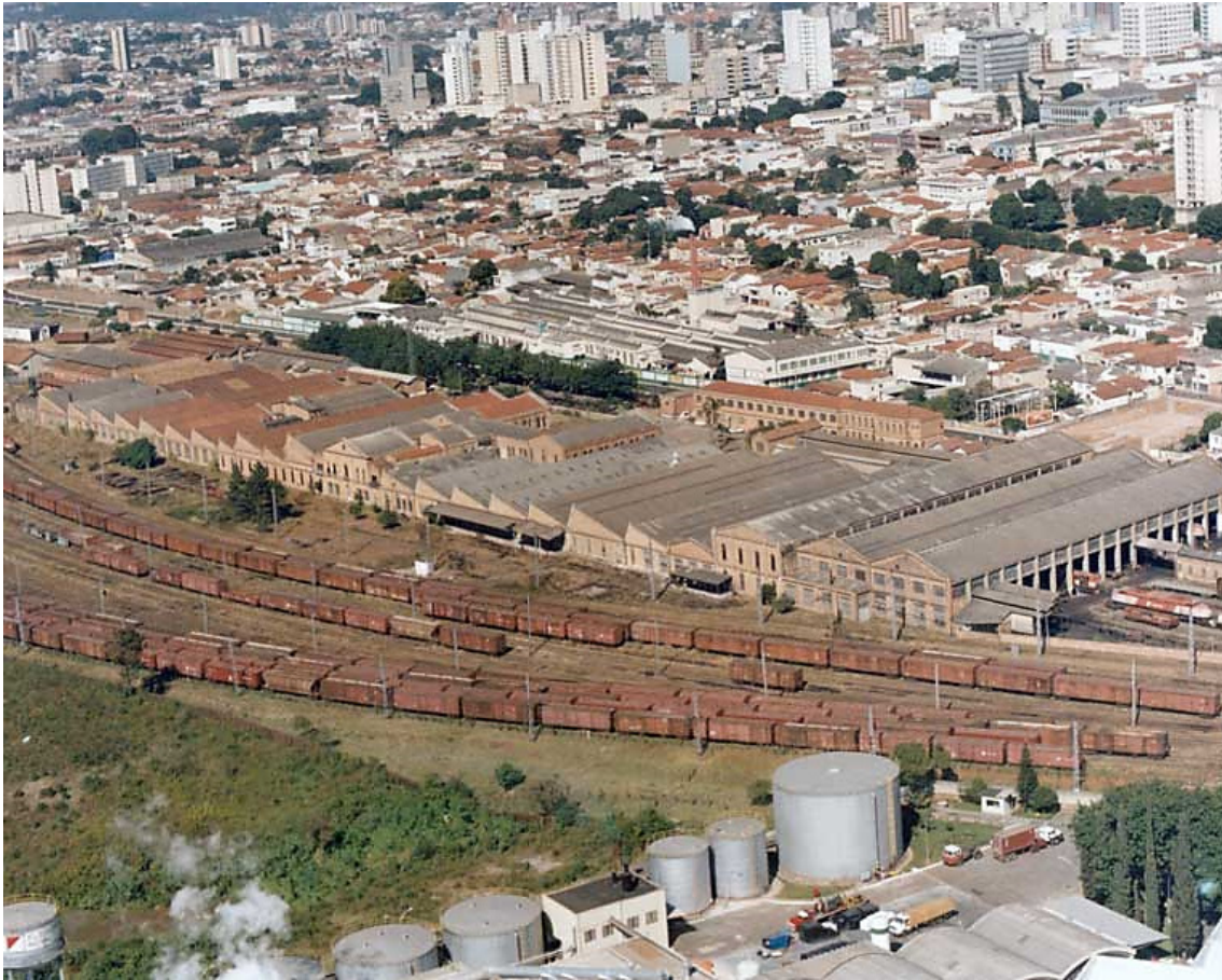
Fig. 11 Complex of the Jundiaí workshops in 1992.
