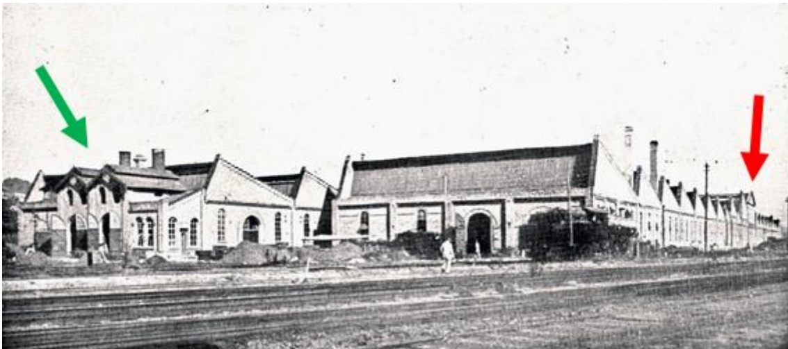
Fig. 3 View of Jundiaí workshops from the railway line. The red arrow indicates where the Inspection Department of the company worked. The green arrow shows the original features of the workshops before the expansion taking place in the 1950s.
