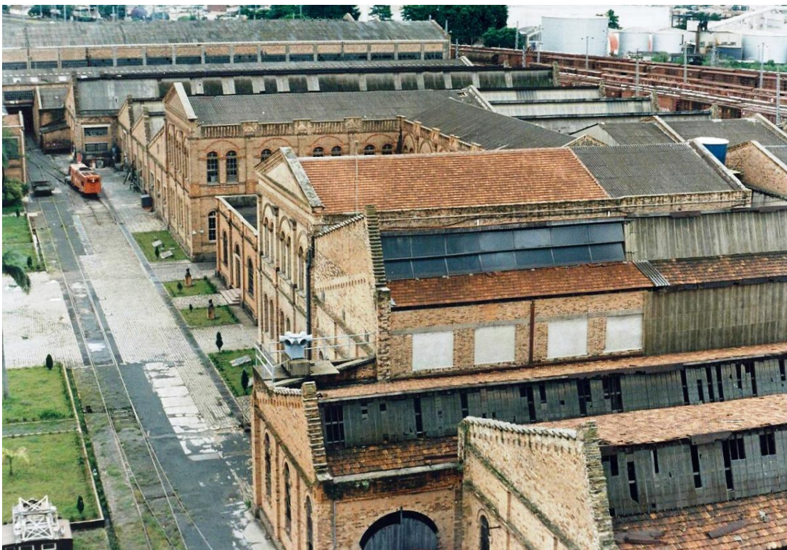
Fig. 10 Aerial view showing the stretch expanded in the 1950s. Note the change in roofing, originally in French tile. Changes like this were probably made during the buildings maintenance work. At the back, the rear view of the workshop built to deal with the diesel-electric units (photo 1999).
