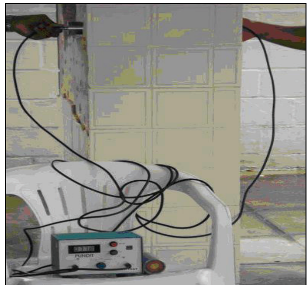
Fig. 2 Test speed of the ultrasonic pulse on Column P1 of Building A.
