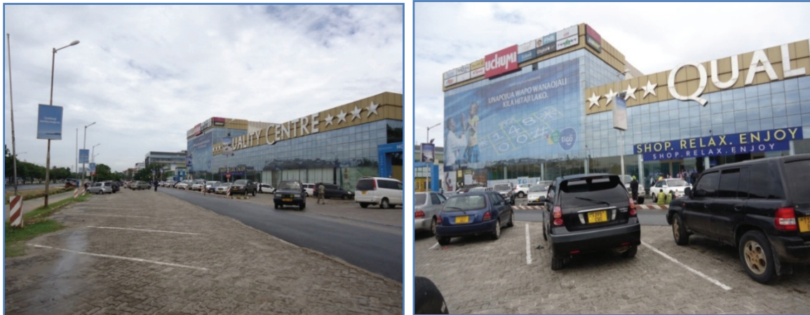
Fig. 2 Quality Centre shopping mall.
