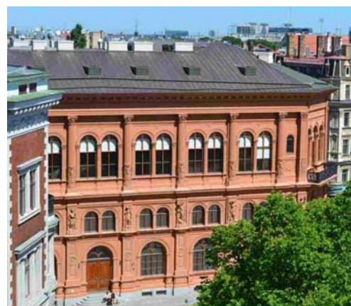
Fig. 1 The Riga bourse building after restoration.
