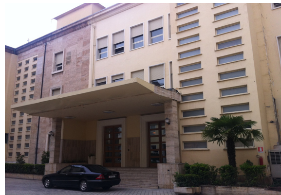
Fig. 1 View of the structure.
