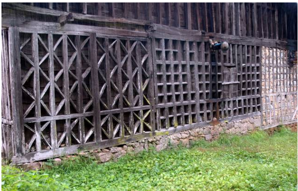
Fig. 12 Detail of filled triangle cell technique.
