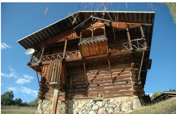
Fig. 5 Usage of wood—timber heap style.
