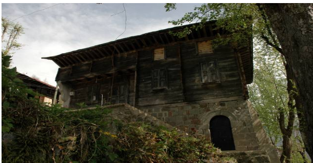
Fig. 7 A house built on a stone masonry ground floor and upper floor is constructed by timber heap technique.
