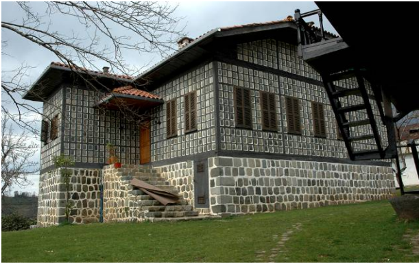
Fig. 9 A house constructed with filled cell technique.
