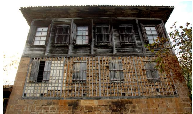
Fig. 6 Usage of stone as a basement wall and filling material.
