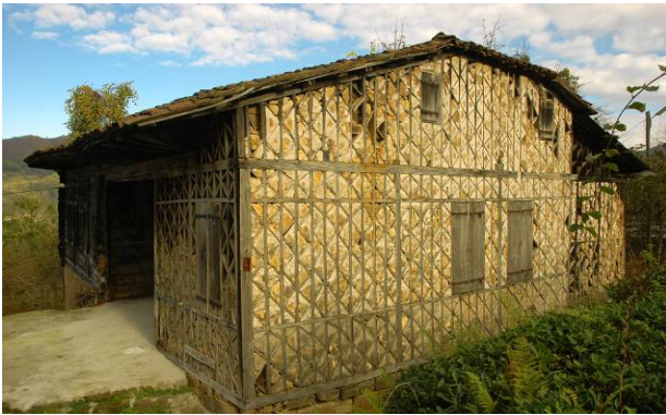
Fig. 11 A house constructed with the technique of filled triangle cell.
