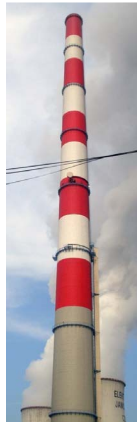
Fig. 2 The industrial chimney located at the power plant Jaworzno III.
