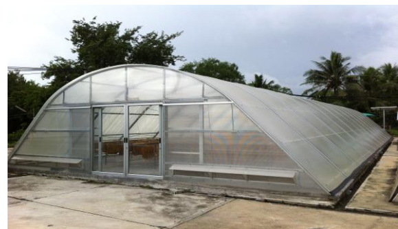
Fig. 1 The pictorial view of the large-scale greenhouse solar dryer.
