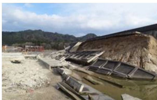
Fig. 14 Slipped off tide wall (No. 4).
