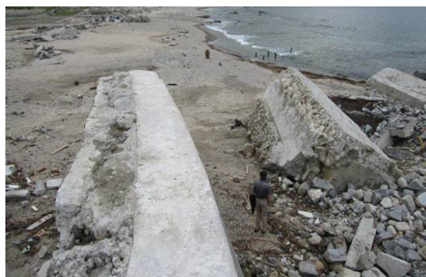
Fig. 13 Damage to tide wall (No. 8).
