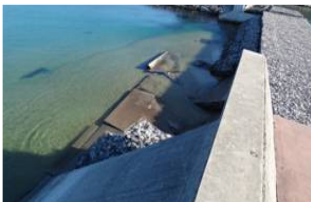
Fig. 17 Damage to tide wall (No. 10).
