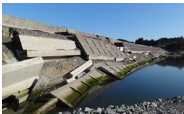
Fig. 16 Slipped off tide wall (No. 10).
