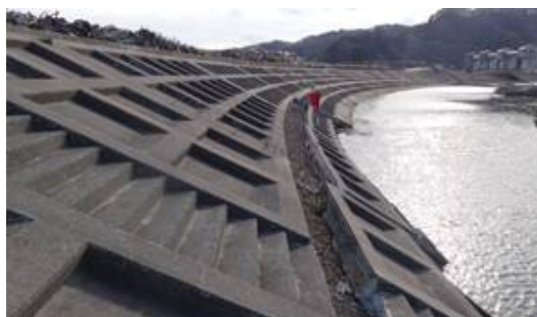
Fig. 11 Slipped off tide wall (No. 6).
