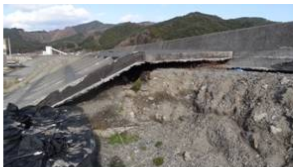
Fig. 10 Damage to tide wall (No. 6).
