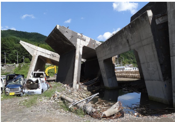
Fig. 22 Damage to tide wall (No. 7).
