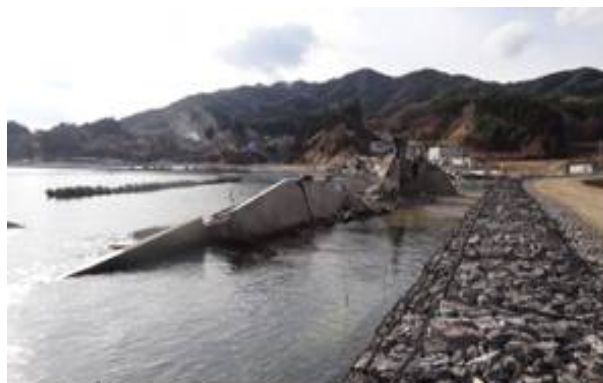
Fig. 15 Damage to tide wall (No. 4).
