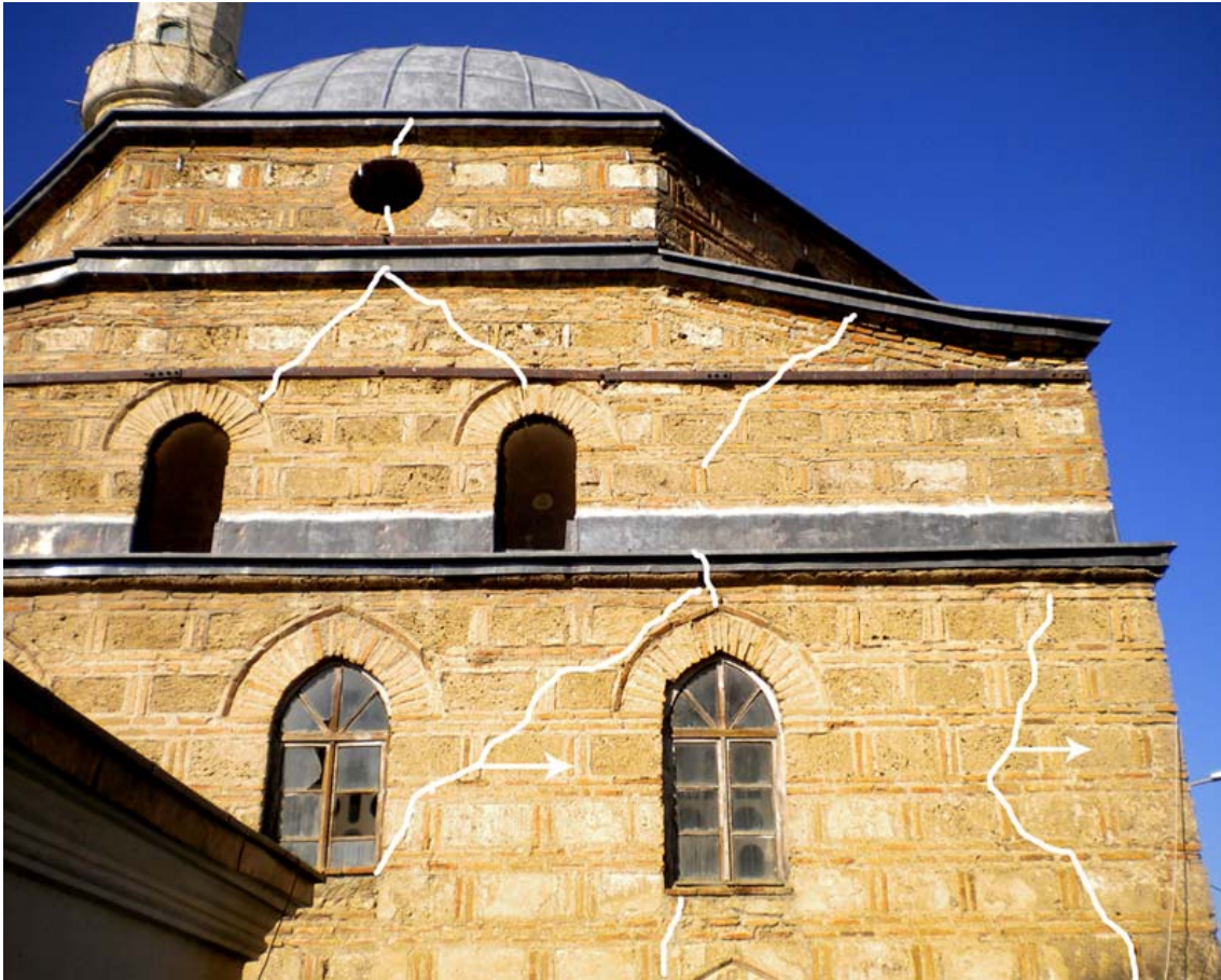
Figure 5. Cracks on the load bearing walls in the south facade of the mosque.
