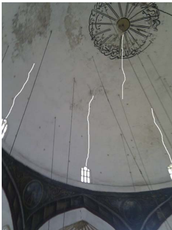
Figure 4. Cracks on the dome and spall of plaster.
