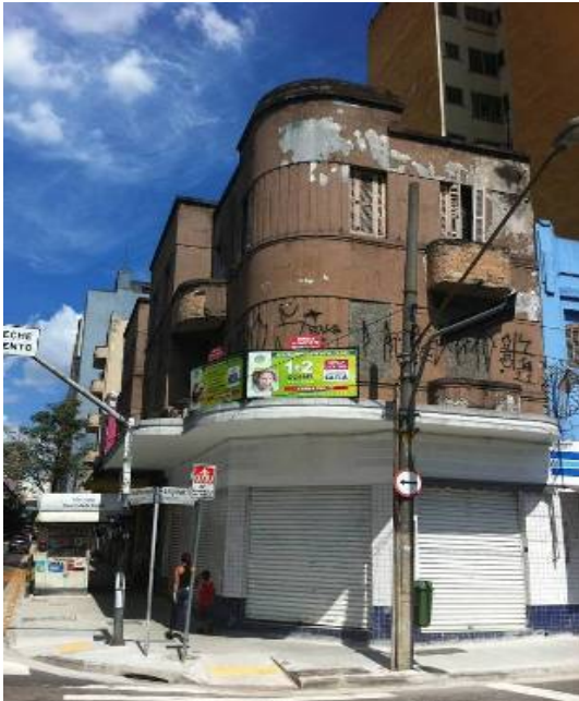
Fig. 1 Building to be rehabilitated released by the real estate market in São Paulo's downtown.
